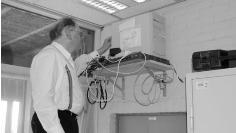
Figure 4.5: Deconstructing a node for replacement
