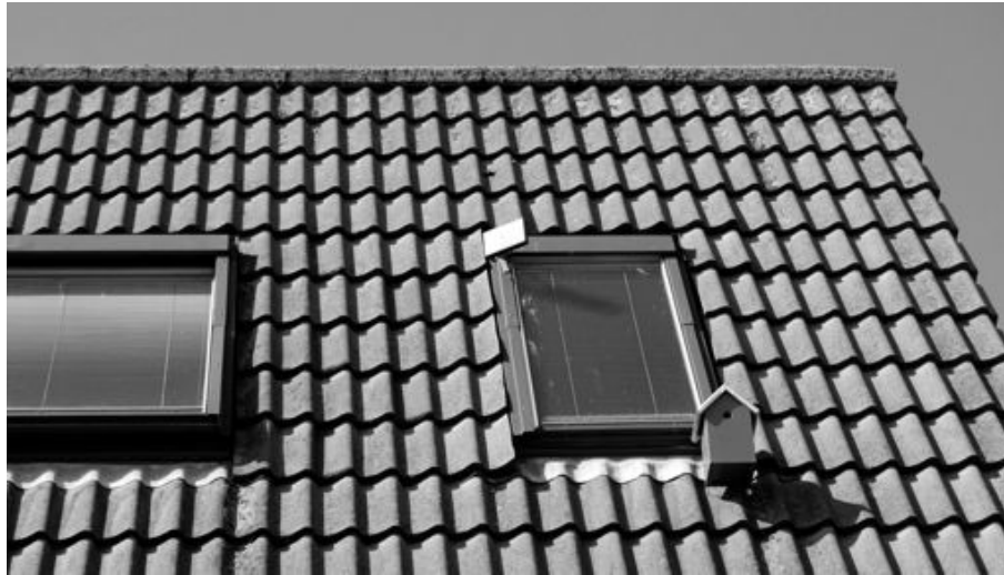
Figure 3.6: Ad's unobtrusive antenna placed in the left upper corner of the skylight
